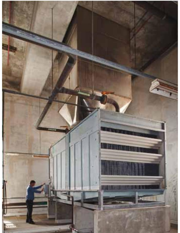
Super sized – one of three cooling towers, fitted with a variable-speed drive to reduce power consumption. Photocall Image Management.
